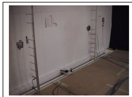
Figure 1 The measurement set-ups with wall convectors (left) and underfloor convectors (right)
